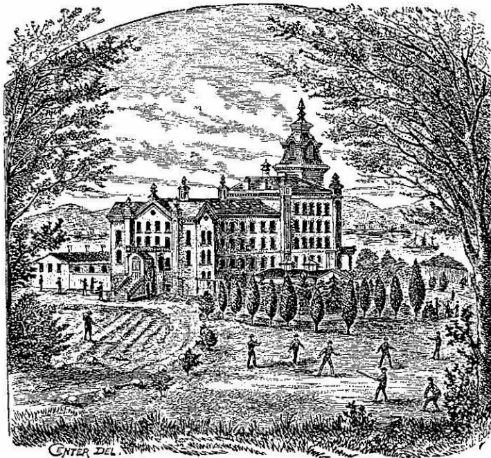
VIEW FROM ENTRANCE OF PARK GROUNDS.
